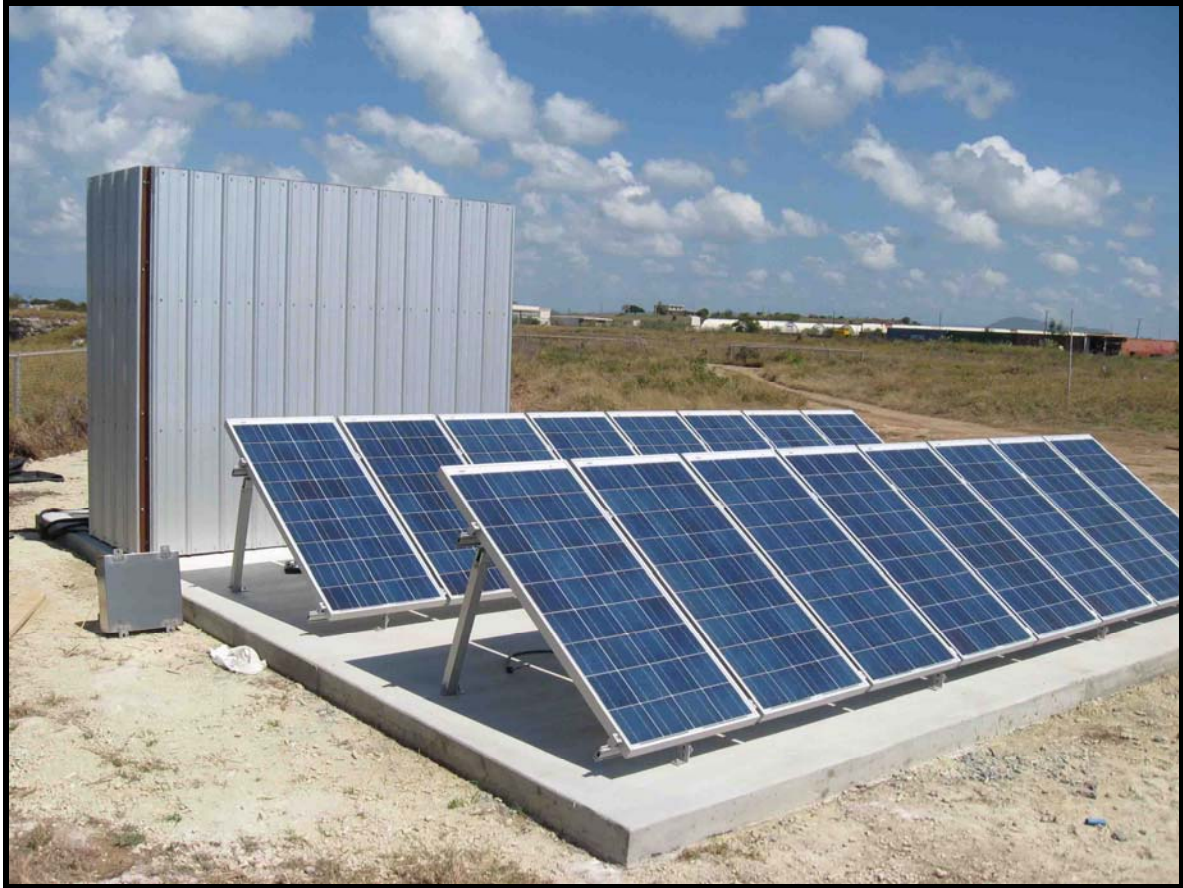
Concrete Slab Mount
